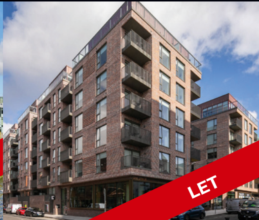
One Lime Street, Dublin 2.
